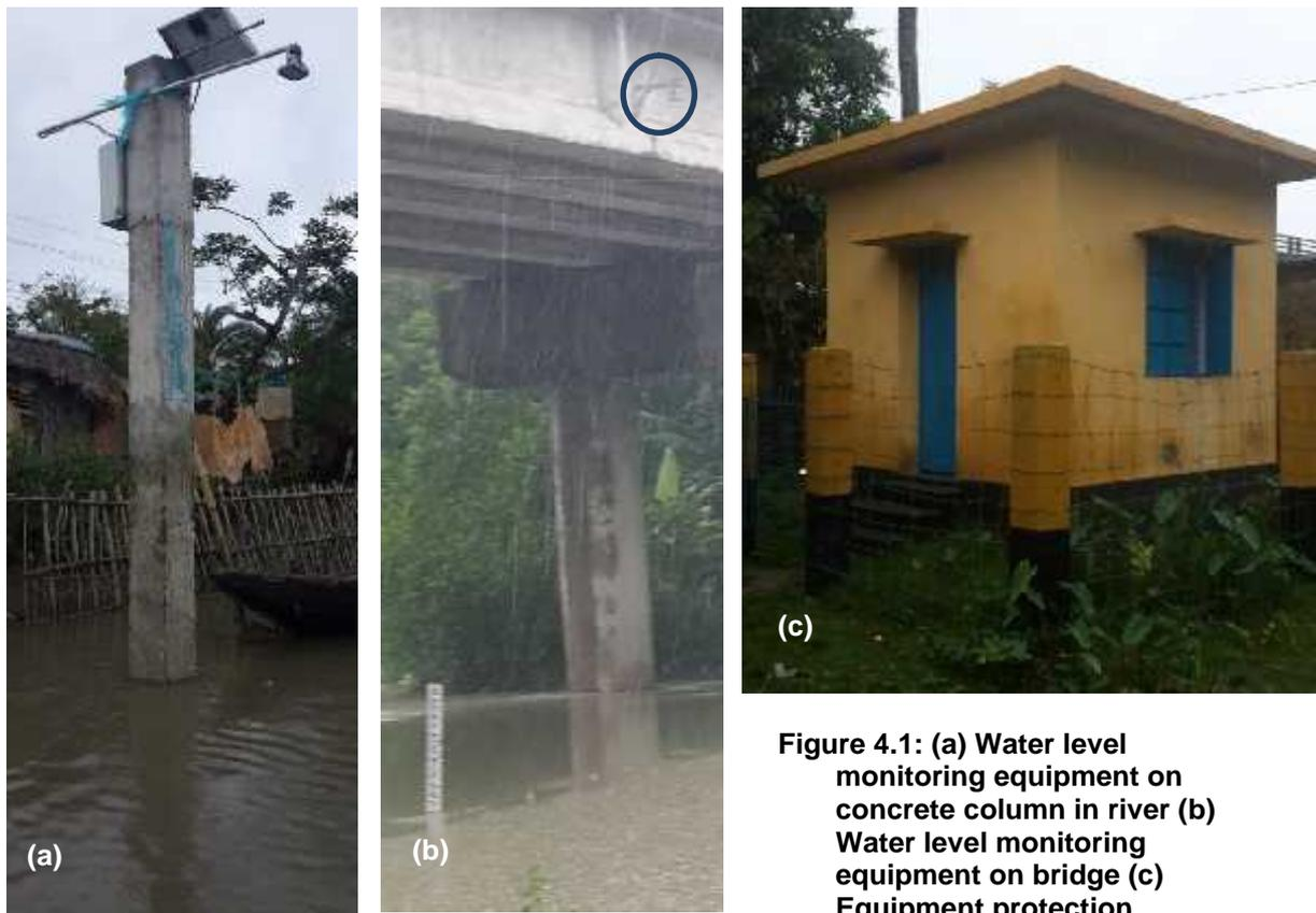
**Figure 4.1: (a) Water level monitoring equipment on concrete column in river (b) Water level monitoring equipment on bridge (c) Equipment protection structure**
