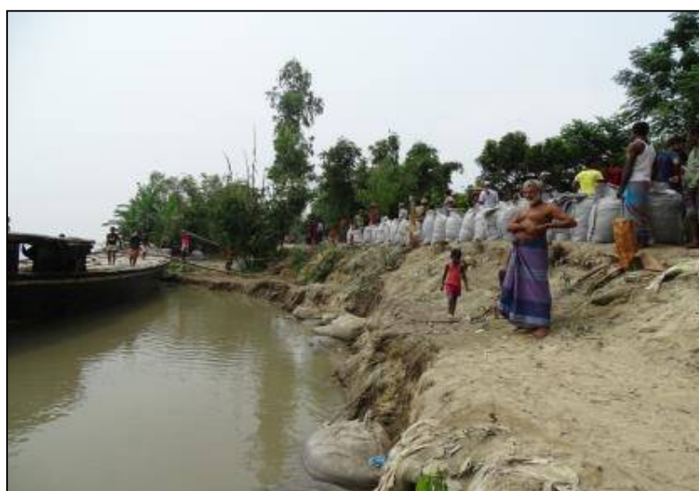
Figure 7.1: River Bank Erosion along Jamuna
