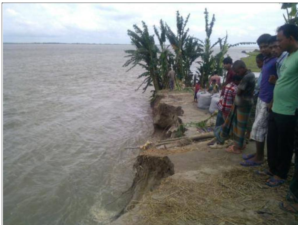
Figure 9.3: Riverbank Erosion near Chandanbaissa
