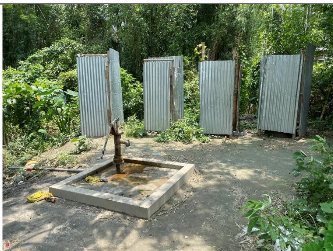
16. Toilets found to be constructed too close to tube well, which poses a significant health risk to the labourers. The Contractor was instructed to clearly mark these tube wells as 'Not For Drinking Water' and provide an alternative supply
