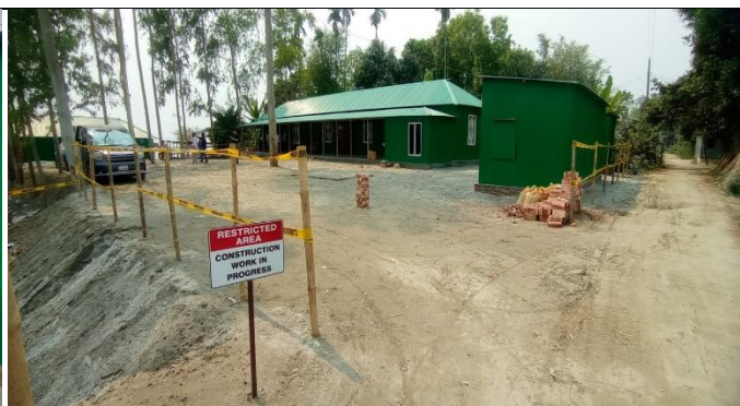
10. Site office fencing with safety signboard.
