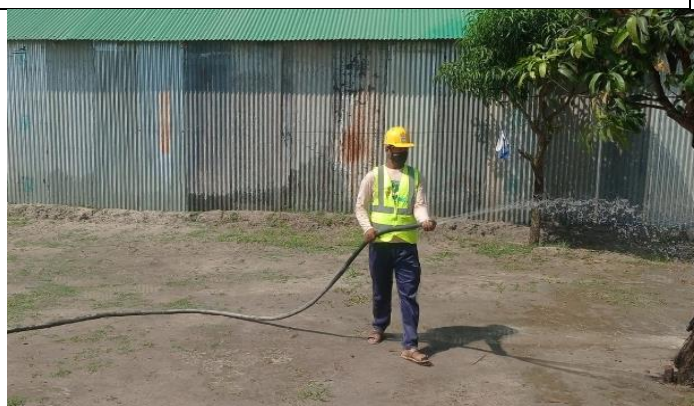
12. Spraying of water for dust suppression
