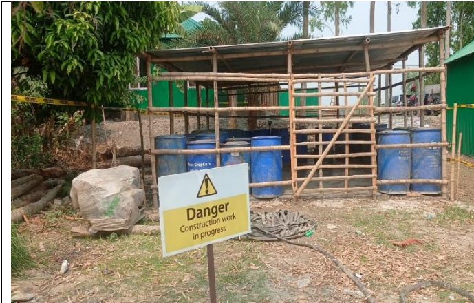
1. Fuel and lubricant were placed on concrete surface.
