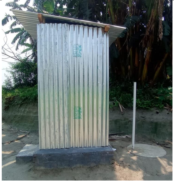
4. Hygienic toilets with sock pit for visitors.
