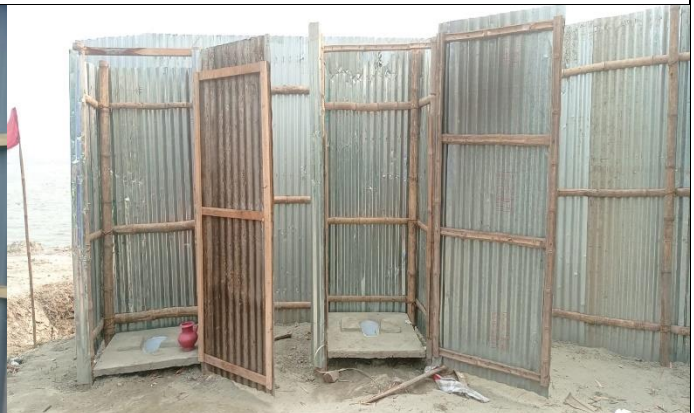
4. Toilets for labors.
