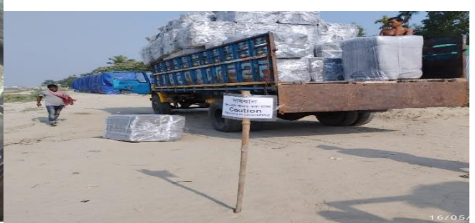
14. Traffic management signboards.
