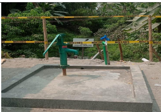
16. Toilets found to be constructed too close to tube well, which poses a significant health risk to the labourers. The Contractor was instructed to clearly mark these tube wells as 'Not For Drinking Water' and provide an alternative supply
