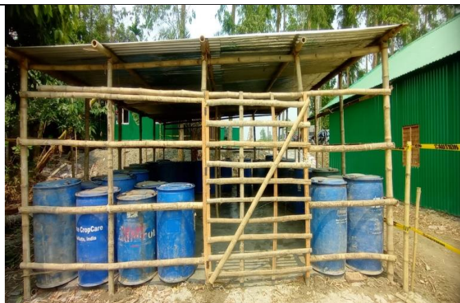
13. Fuel and lubricant were placed on concrete surface and protected roof.
