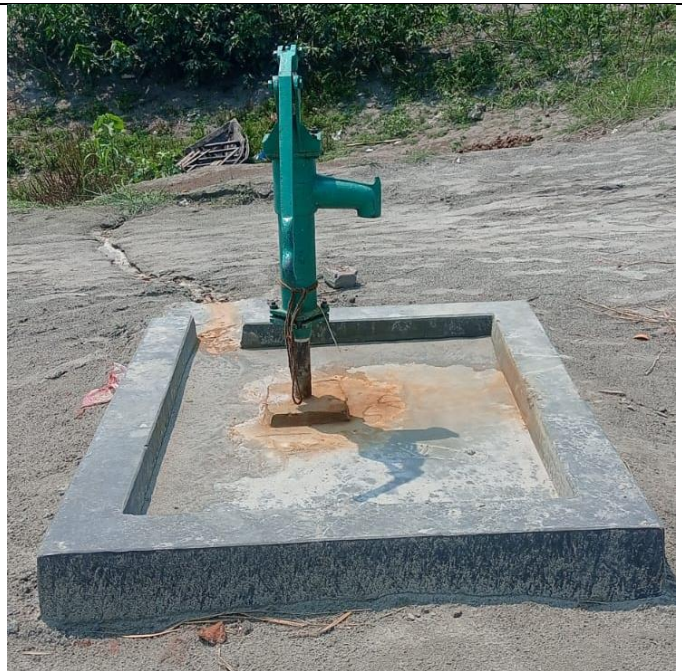
6. Tube well was found with concrete floor and proper disposal system.
